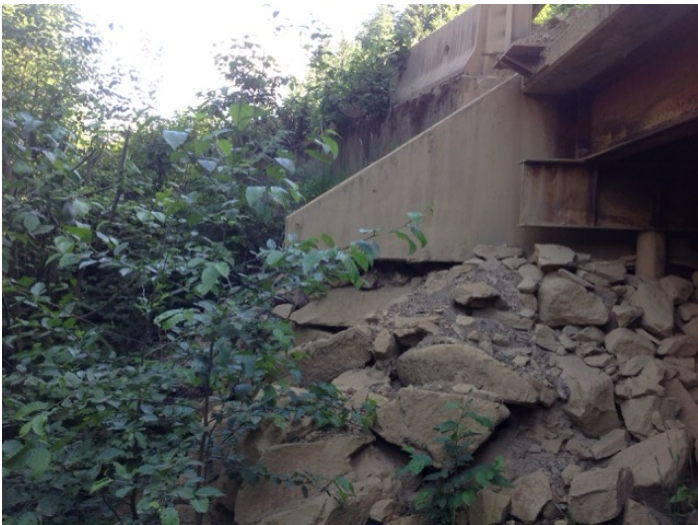
right downstream wall
