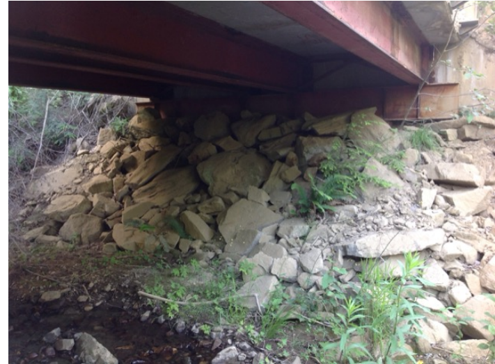
Left Bank Abutment when facing downstream
