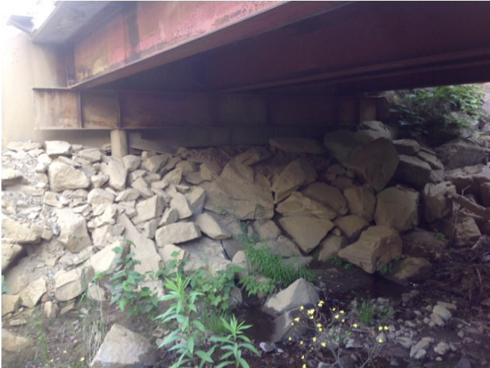
Right Bank Abutment when facing downstream
