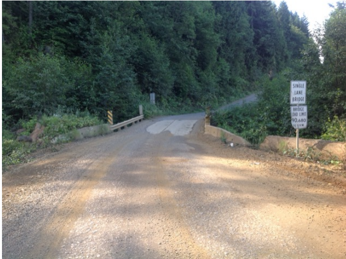
Approach from Right Bank when facing downstream
