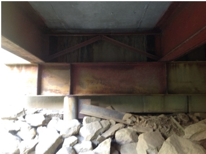
downstream girder set
