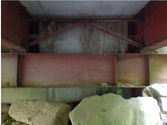
upstream girder set shimmed due to different deck thicknesses
